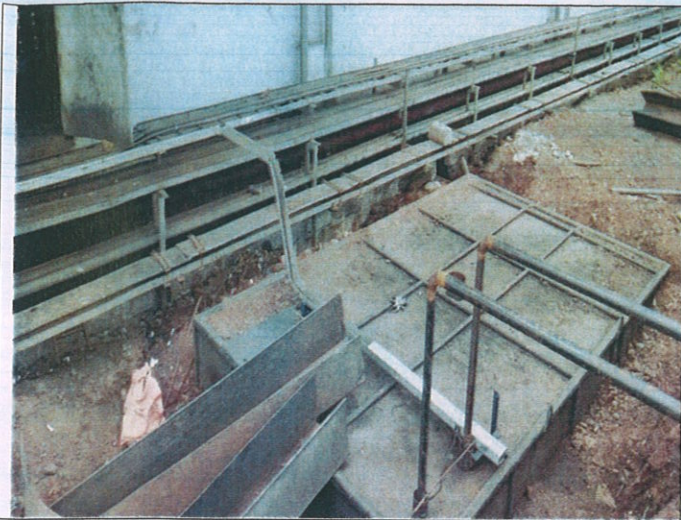
RAINWATER HARVESTING SYSTEM
